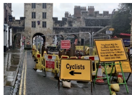
When temporary cycle provision is created it is essential it still meets suitable guidance, such as the 1.5m width requirements
