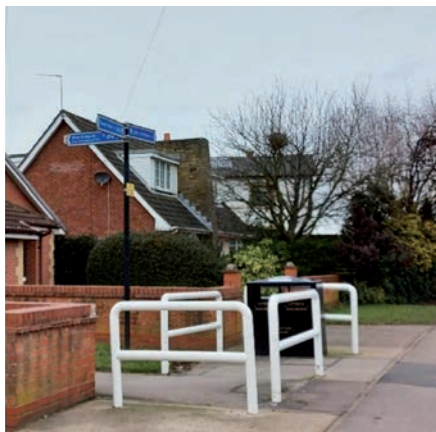
New Lane to Stafford Way cycle path to avoid busy roads/junction. Inaccessible due to offset barrier (worsened by dog waste bin placed inside barrier)
