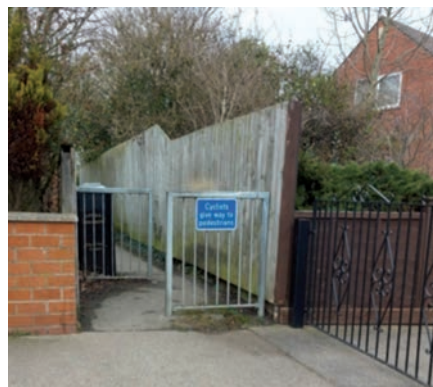
Offset barrier/chicane preventing access from Straylands to Malton Road (to avoid busy junction)
