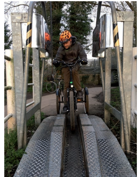
A tricycle attempting to negotiate the bespoke footplates installed at one of the entrances to Hob Moor
